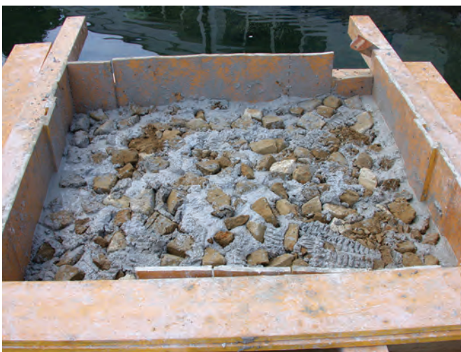
Fig. 5.20. Final upper surface of the concrete within the formwork.
