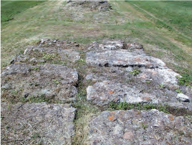
Fig. 8.38. Impression of horizontal tie beams on Molo Sinistro of the Claudian basin at Portus.
