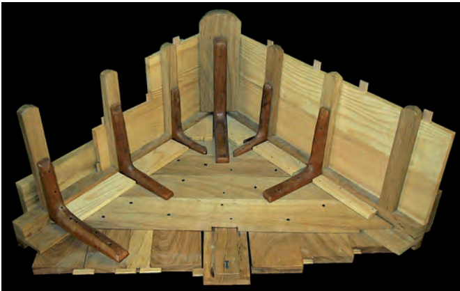
Fig. 8.56. Model of the bow section of the caisson used to construct the bridge pier at Chalon-sur-Saône (C. J. Brandon).
