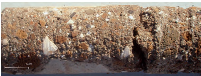
Fig. A3.52: CHR.2007.02, -0.40 to -0.65 m. Porous mortar with a high proportion of pale orange pumiceous pozzolan, and angular fragments of poorly calcined limestone.
