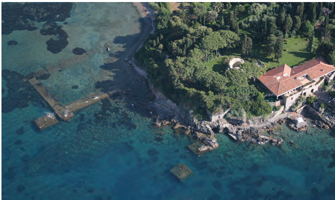
Fig. 4.18. Santa Liberata, aerial photograph of villa, piscina, and pilae (Courtesy of P. Gambogi).
