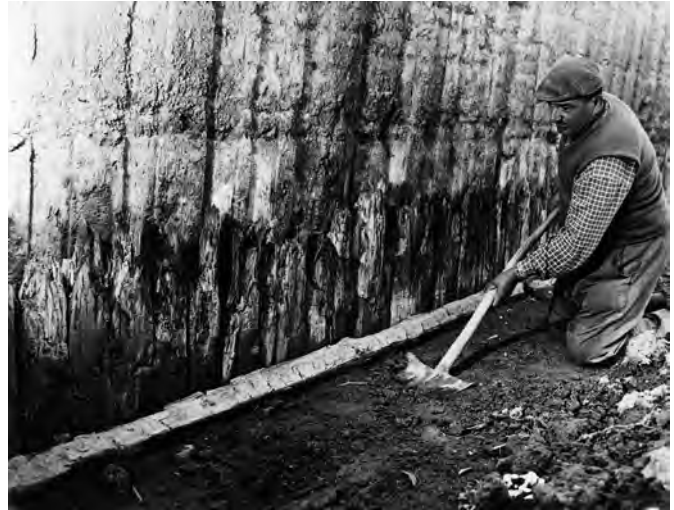
Fig. 8.23. Remains of the lower section of formwork on the northern mole at Portus (O. Testaguzza, used with permission).
