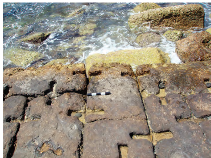
Fig. 4.49. Pompeiopolis, detail of clamp recesses on west breakwater.
