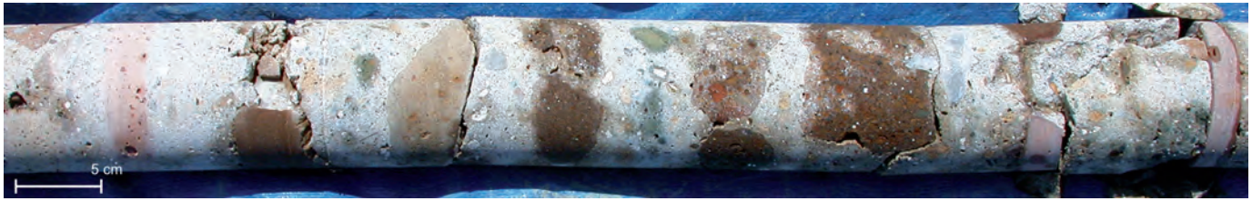
Fig. A3.24: PTR.2002.01, detail -0.42 to -1.16 m. Tufo Lionato and ceramic caementa, and a well-consolidated mortar with gray pumiceous ash pozzolan.
