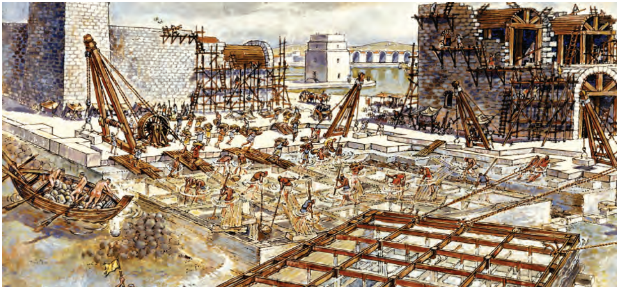
Fig. 5.10. Reconstruction of workers lowering mortar into formwork at Sebastos (Hohlfelder 1987: 264–65) (National Geographic Society, used with permission).
