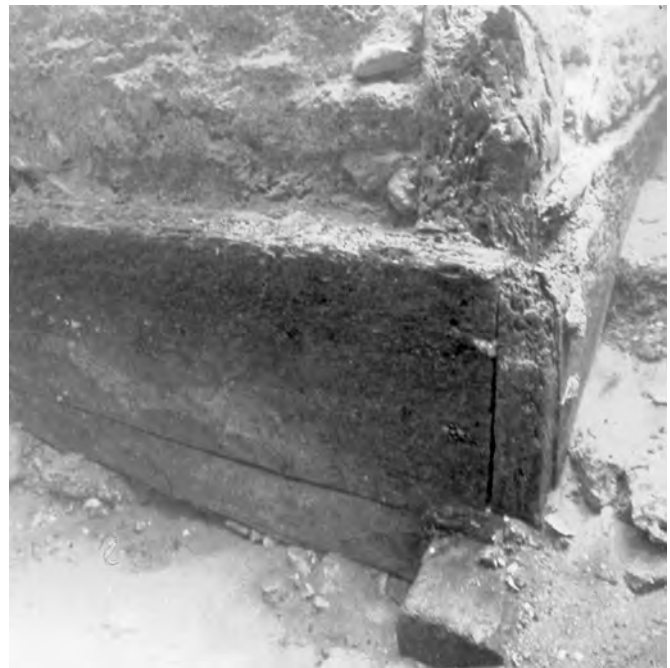
Fig. 8.69. Corner of caisson K-3, Caesarea (A. Raban).
