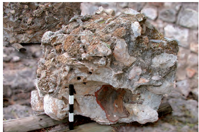
Fig. 6.3. Two fragments of concrete wall from the Quarteira piscina, now in the Loulé Archaeological Museum. The near fragment is a cross-section showing the use of an embedded amphora body as a nesting pot.
