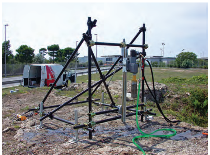
Fig. 3.16. Frame constructed of iron scaffold tubes.
