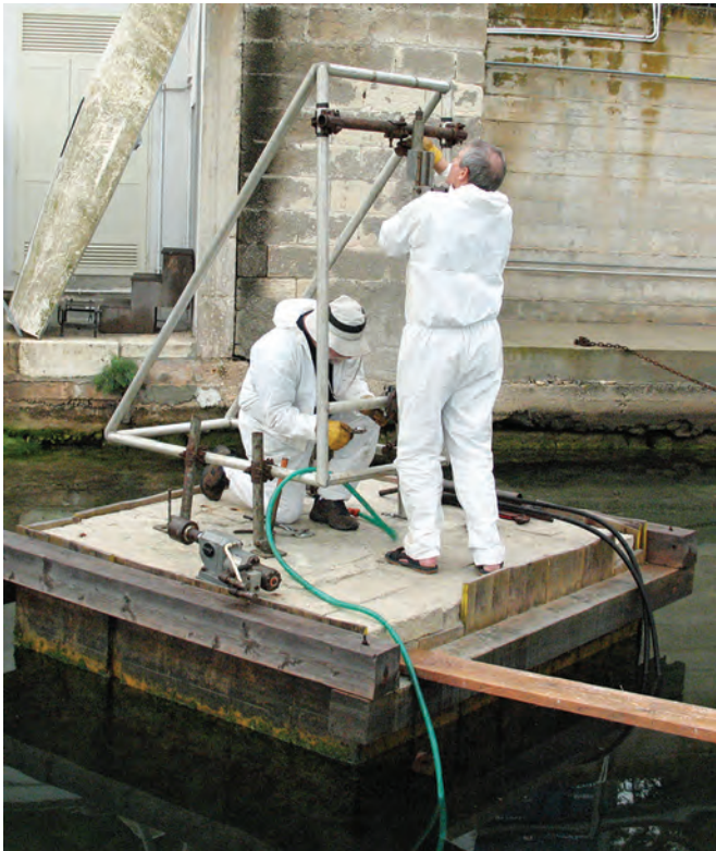
Fig. 3.17. Cordiam M60 rack clamped to purpose-made aluminium frame.
