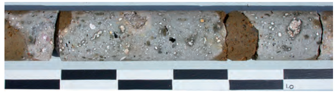
Fig. A3.9: PCO.2003.01, detail, -0.50 to -1.10 m. Pumiceous tuff caementa and pumiceous mortar with abundant lime clasts.
