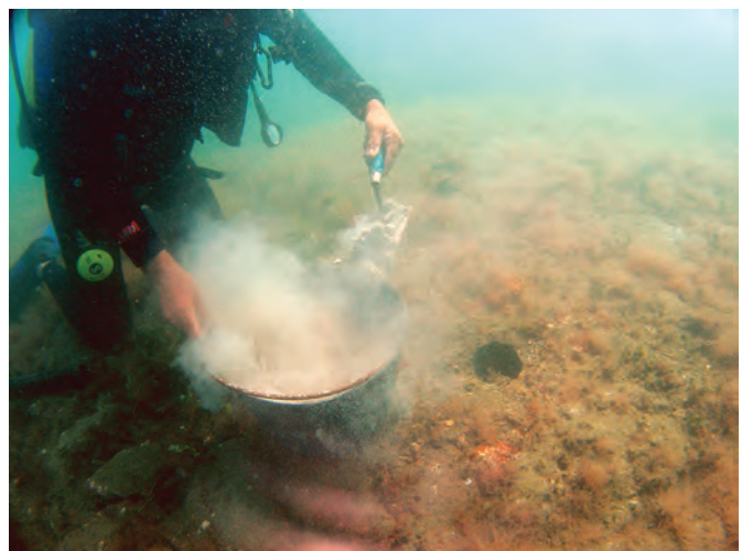
Fig. 3.44. Weak mortar mix being trowelled into core hole.
