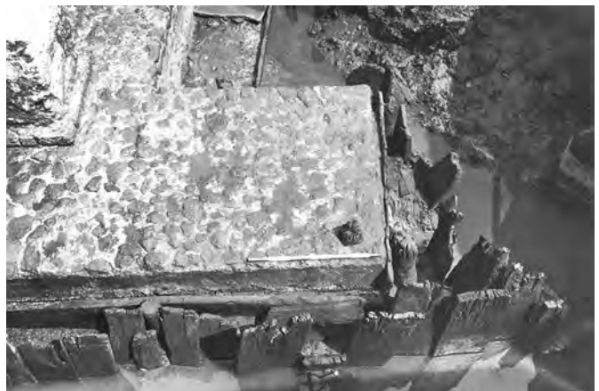
Fig. 8.30. Vertical timber retaining wall around the concrete platform in front of the Spring House at Cosa (McCann et al. 1987: 101, fig. V.6–V.7) (Photo: A. M. McCann, used with permission).
