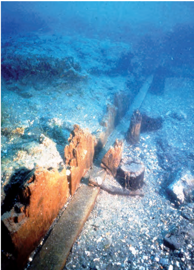
Fig. 8.18. Base of shuttering on the side of a concrete dock south of the Baianus Lacus entrance channel (Scognamiglio 2002: fig. 2; photo E. Scognamiglio).
