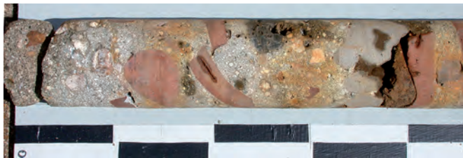
Fig. A3.11: PCO.2003.02, detail 0 to -0.46 m. Ceramic and lava caementa in iron stained concrete, an artefact of the drilling process, and mortar with pale orange pumiceous pozzolan and complex relict lime clasts. Scale bar is 10 cm.
