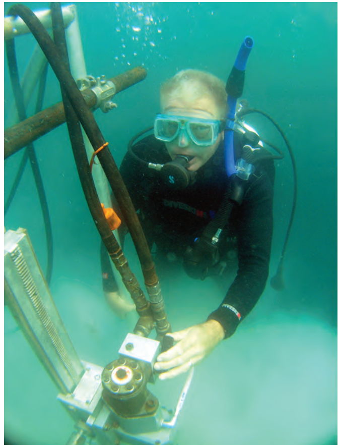
Fig. 3.21. Twin hydraulic hoses connected to the drill motor unit.
