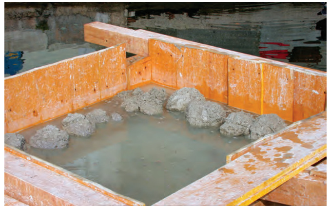
Fig. 5.17. Basket loads of mortar visible in shallow water in formwork.
