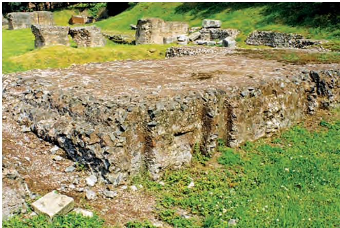
Fig. 8.1. Formwork impressions on a concrete foundation on the Palatine Hill, Rome.
