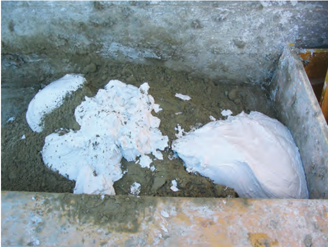
Fig. 5.8. Pozzolana and lime putty in the mixing trough.
