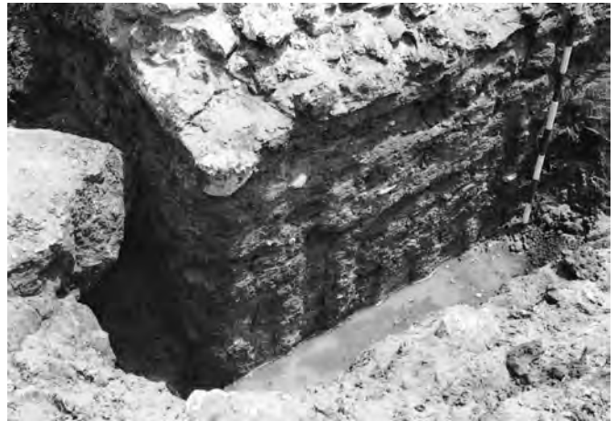
Fig. 4.12. Portus Cosanus, impressions of wooden formwork shuttering on Pier 1 (after McCann et al. 1987: fig. III–13). (Courtesy of A. M. McCann)
