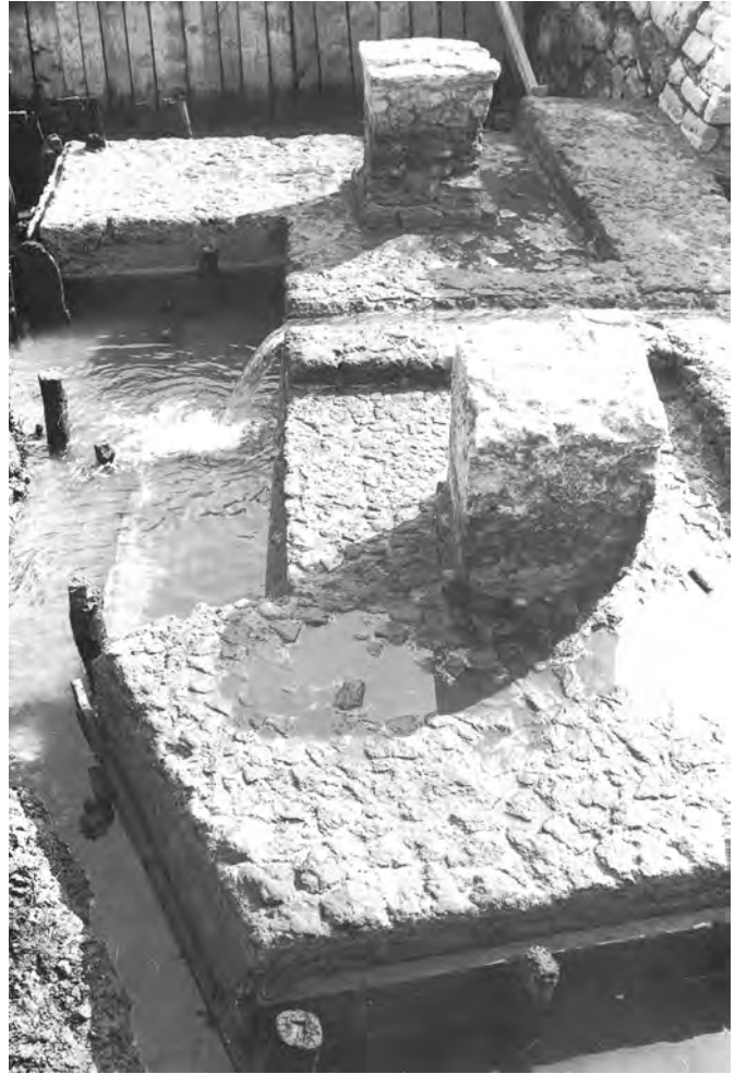
Fig. 8.29. Horizontal planked formwork around the platform in front of the Spring House at Cosa (McCann et al. 1987: 100–1, fig. V.4–V.12) (Photo: A. M. McCann, used with permission).
