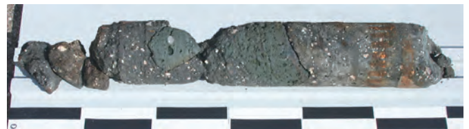
Fig. A3.18: PCO.2003.05. Overview of highly weathered concrete core, with pumiceous tuff caementa and mortar altered to dark green earthy fabrics. Iron staining is an artefact of the drilling process.
