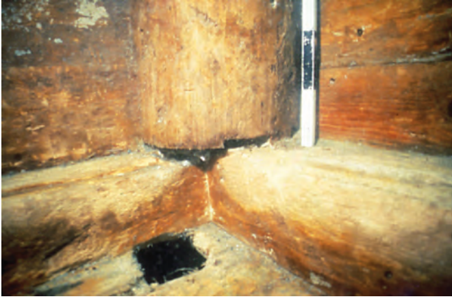
Fig. 8.74. Detail of the corner of the inner cell within caisson K-2, Caesarea (A. Raban).
