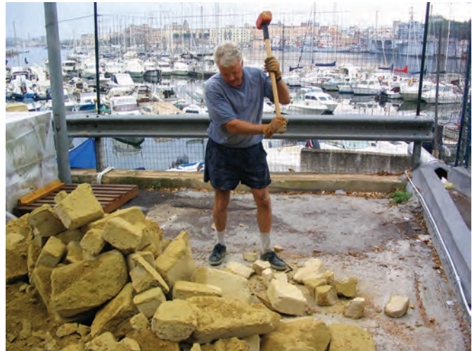
Fig. 5.5. Tuff blocks being reduced to caementa for the pila reconstruction.
