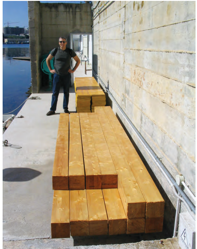
Fig. 5.3. Reconstituted lumber ready for use in the formwork.
