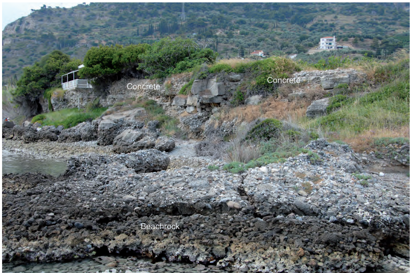
Fig. 6.63. Mavra Litharia , natural beachrock formation with raised concrete wall in background.
