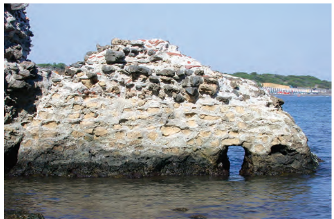
Fig. 4.14. Portus Cosanus, seaward portion of Pier 2, showing upper and lower concrete mixtures and hole left by catena.
