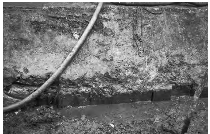
Fig. 8.35. Remains of vertical timber planking shuttering at the southwest corner of the Darsena basin at Portus (Verduchi 2005: 257; used with permission).
