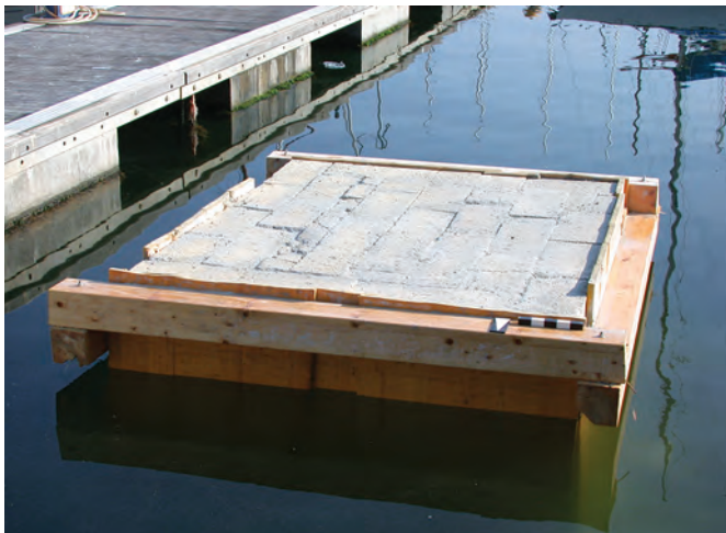
Fig. 5.21. Completed pila with paved upper surface.
