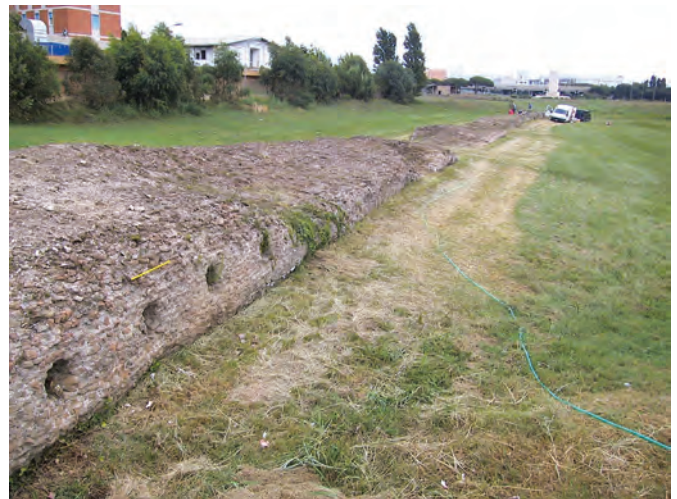
Fig. 4.3. View of eastern end of Molo Sinistro, with sockets left by formwork. Site of POR.2002.01 in foreground, POR.2002.03 in background.
