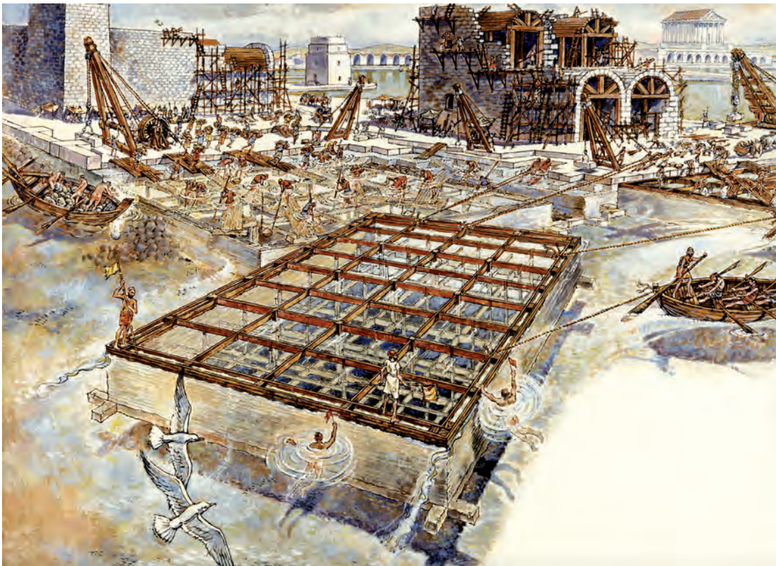
Fig. 8.61. Reconstruction of floating formwork being manoeuvred into position over Area G at Sebastos (Hohlfelder 1987: 264–65) (National Geographic Society, used with permission).
