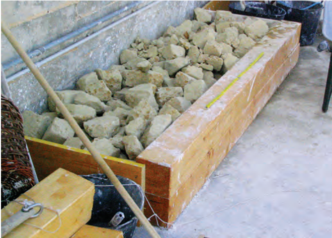
Fig. 5.18. Trough filled with measured volume of tuff caementa.
