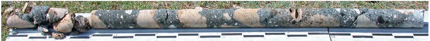
Fig. A3.66: CAE.2005.05. Overview of sea-water saturated core, calcareous sandstone caementa , occasional small pumiceous tuff clasts, and mortar with relict lime. Scale bar is 10 cm.
