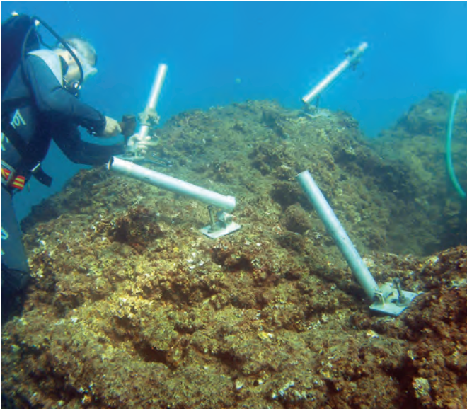
Fig. 3.38. Frame feet being fixed to an uneven concrete surface at Caesarea.
