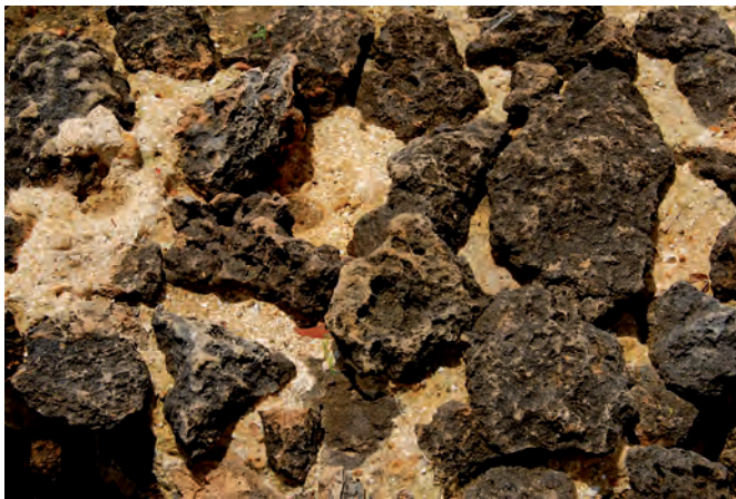
Fig. 6.81. Carthage, Neptune block, detail of concrete.
