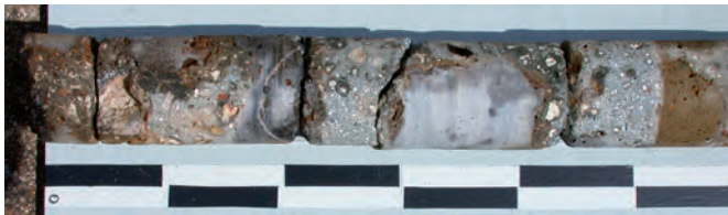
Fig. A3.8: PCO.2003.01, detail, 0 to -0.58 m. Pumiceous tuff and gray limestone caementa , and mortar with relict lime clasts and possible clots of relict lime putty.
