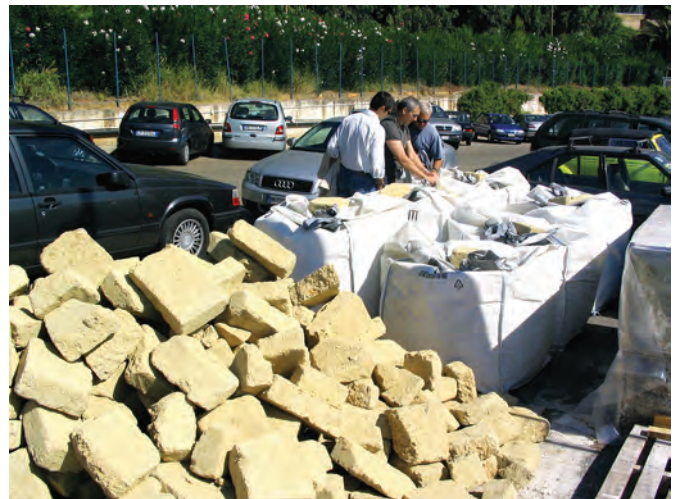
Fig. 5.2. Tuff blocks and bags of pozzolana assembled for the reconstruction project.
