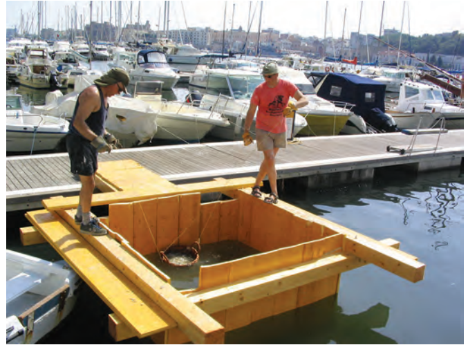
Fig. 5.15. Basket of mortar floating in the inundated form.
