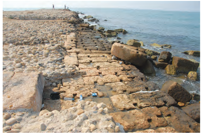
Fig. 4.48. Pompeiopolis, detail of outer wall of west breakwater.
