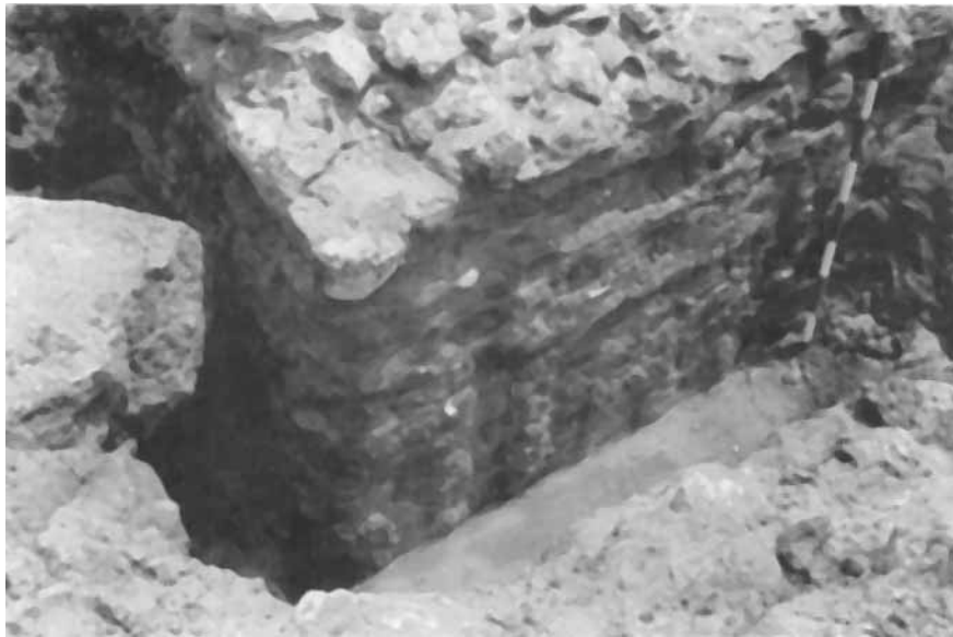
Figure 1. Cosa: impression of vertical board shuttering on Pier 1. Photo: A. M. McCann.
