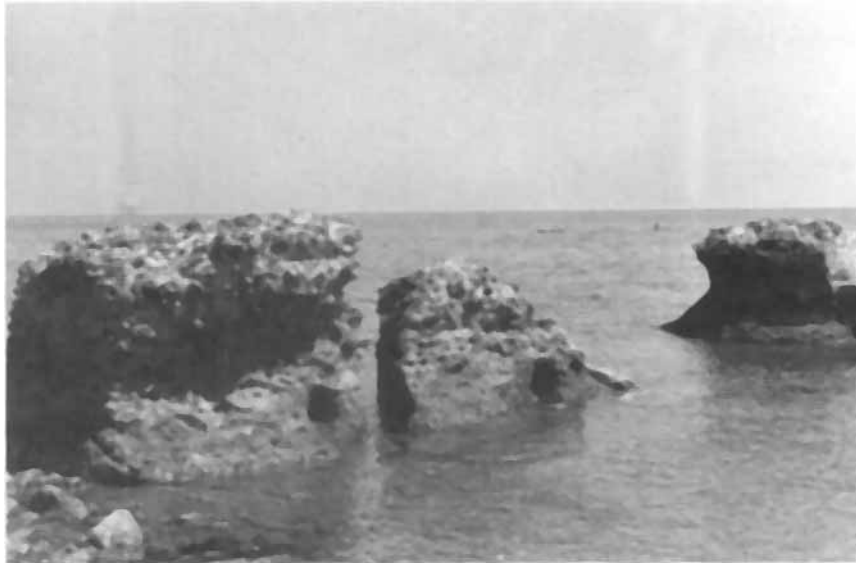
Figure 2. Cosa: holes left by tie beams in Pier 2. Photo: A. M. McCann.
