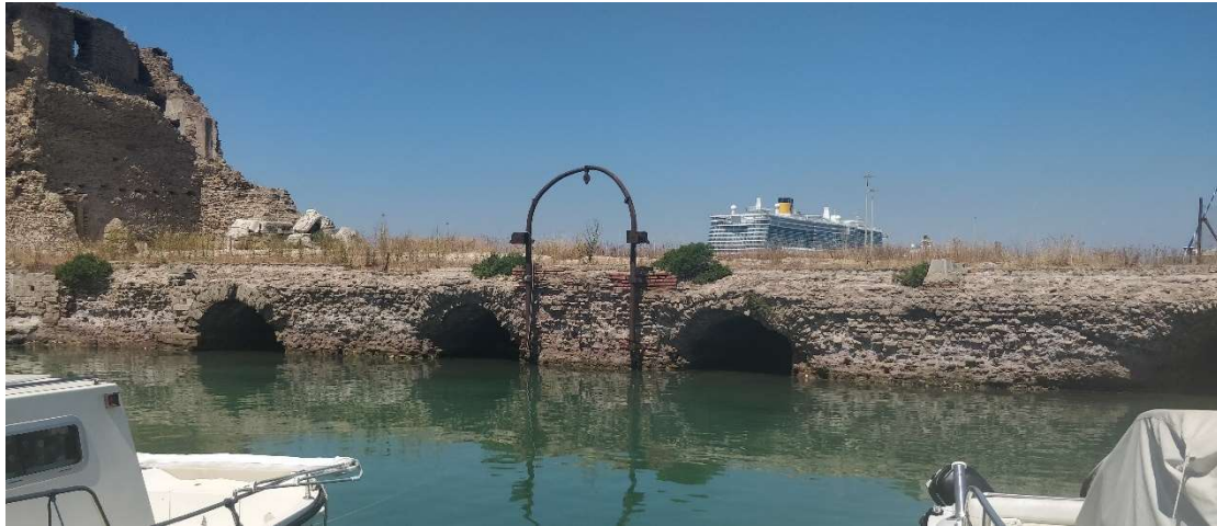
Figure 12. Molo del Lazzaretto at Civitavecchia (Italy). (Photo de Graauw, 2022)
