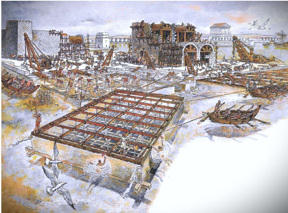
Figure 10. Roman wooden floating caisson with divers, tugs and heavy hoisting equipment, at Caesarea Maritima. (Aquarelle by Robert Teringo, 1987, National Geographic, 171-2)
