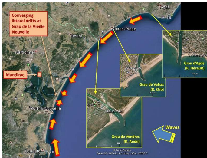
Figure 25. Coastal cell from Leucate to Agde (ca. 55 km) with 3 main river outlets. (Google Earth)
