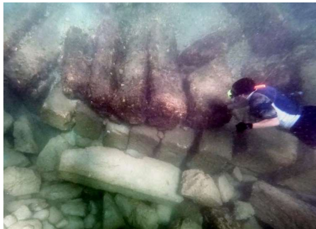
Figure 8. North breakwater of Tyre (Lebanon) built with ashlar headers, (800 BCE). (Photo Goiran, 2019)
