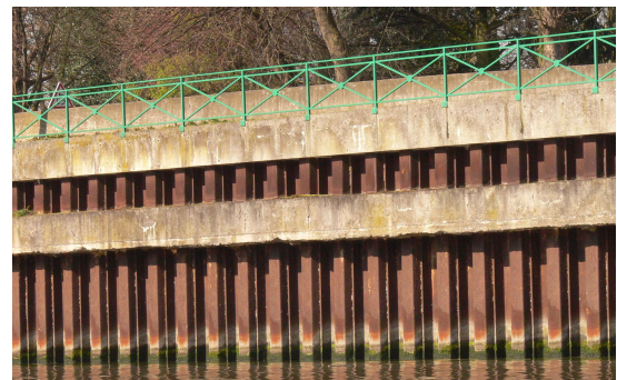
Fig. 31. Steel sheet-piling with heavy concrete capping beam and anchoring beam (Wikipedia)
