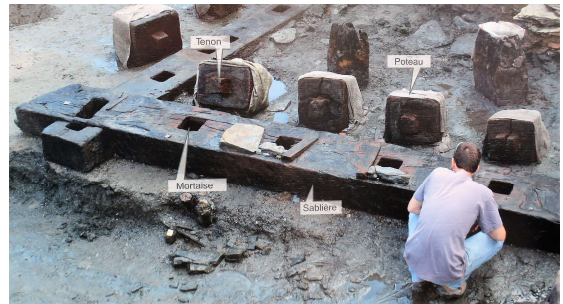
Fig. 29. River quay at Rézé showing connection between lower beam and piles (Mus. Le Chronographe, 2018)
