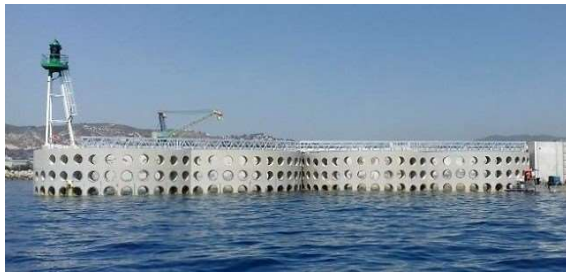
Fig. 14. Jarlan-type wave absorbing caisson
