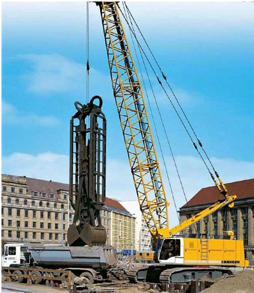
Fig. 32. Slurry-wall grab fitted on a crawler crane (Liebherr, 2018)
