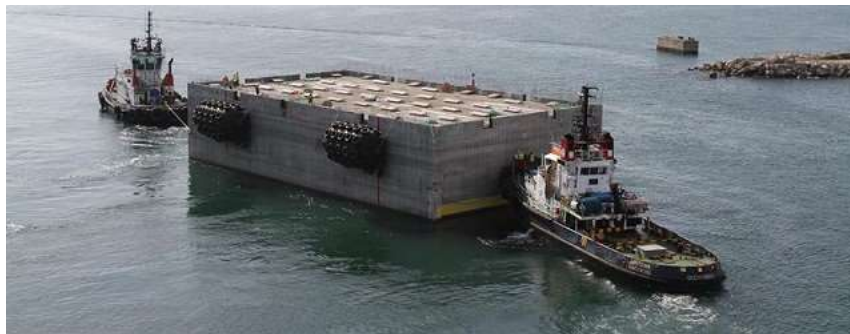
Fig. 13. 45x24x18 m caisson floated into position at Açú (Brazil) (The Corner, 2013)
