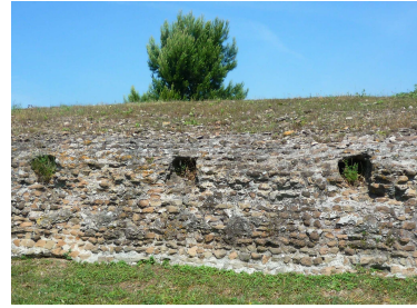
Fig. 6. Portus' north breakwater showing imprints of transverse caisson beams (de Graauw, 2011)
