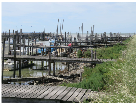
Fig. 24. Small timber jetties at Port du Bec (Goix, France) used by oyster farmers (de Graauw, 2018)
