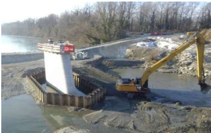
Fig. 35. Cofferdam for bridge pier in river Isère (France) (Eiffage, 2017)
