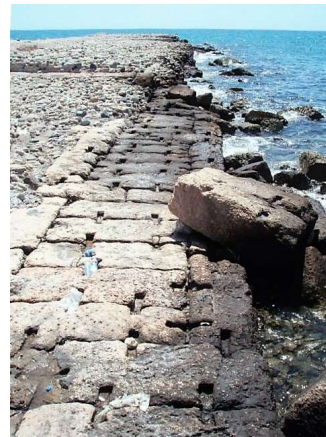
Fig. 9. Marginal ashlar wall (centre) containing marine concrete (left) at Pompeiopolis (Brandon, 2014)
