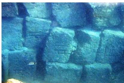
Fig. 3. Tyre north mole built with ashlar headers (0.5x0.5x2 m) (Noureddine, 2010)
