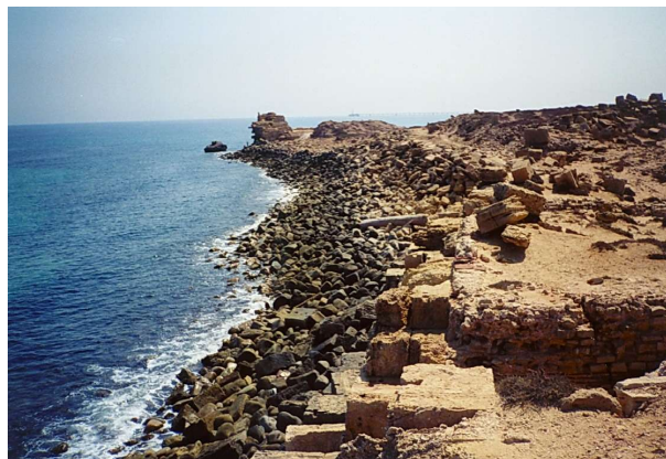
Fig. 39. Berm breakwater on the north coast of Leptis Magna (de Graauw, 2000)
