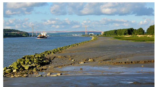
Fig. 45. Typical tidal wetland behind a submersible training wall (GIP Seine-Aval, 2009)
