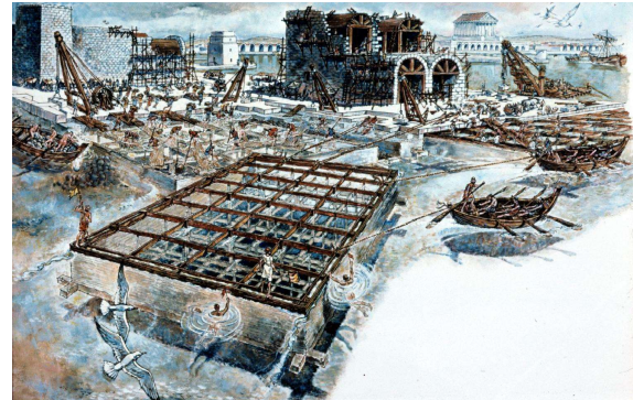
Fig. 7. Reconstruction of a floating caisson being positioned. (J. Robert Teringo, 1987)
