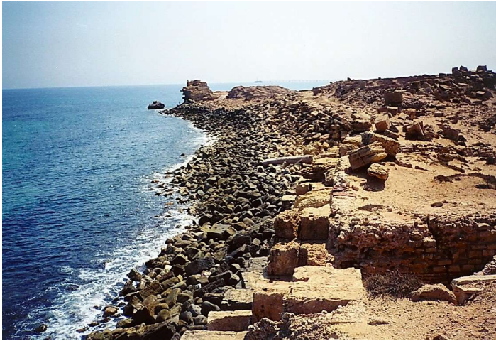
Berm breakwater at Leptis Magna (Photo de Graauw, 2000)
