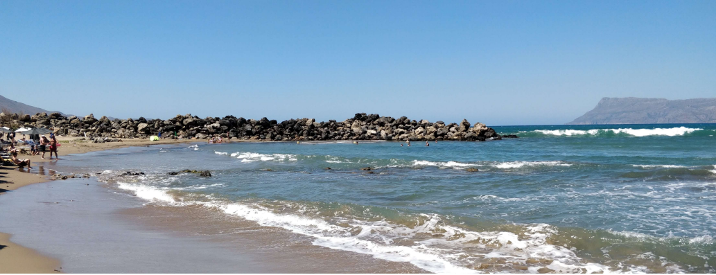
Rubble-mound breakwater at Kissamos (Crete) (Photo de Graauw, 2022)
