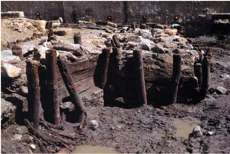
Timber quay wall of place Jules Verne, Marseille (France), (Inrap 1993)
