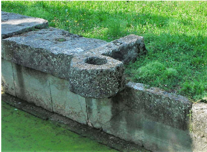
Possible foot-hole of a derrick mast at Aquileia (Italy), (Photo de Graauw, 2010)
