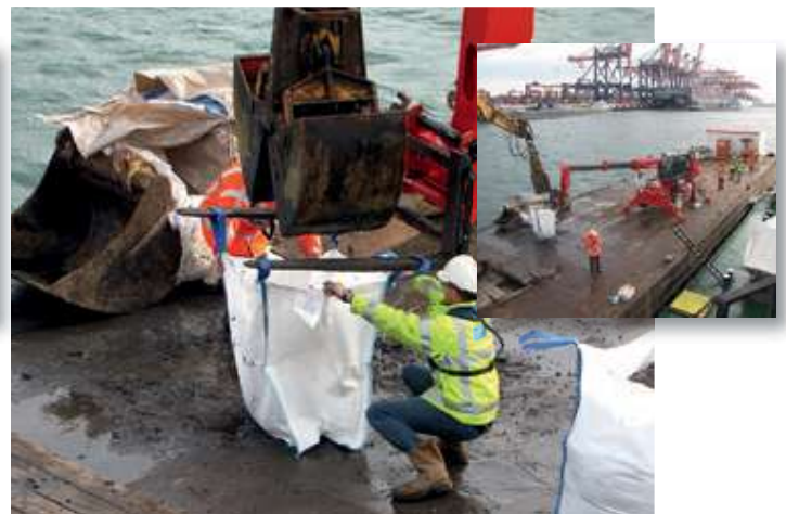
Figure 15. Filling: from receiving container into numbered big bag. Insert, Figure 16. Layout of working pontoon, with storage area at the back.
