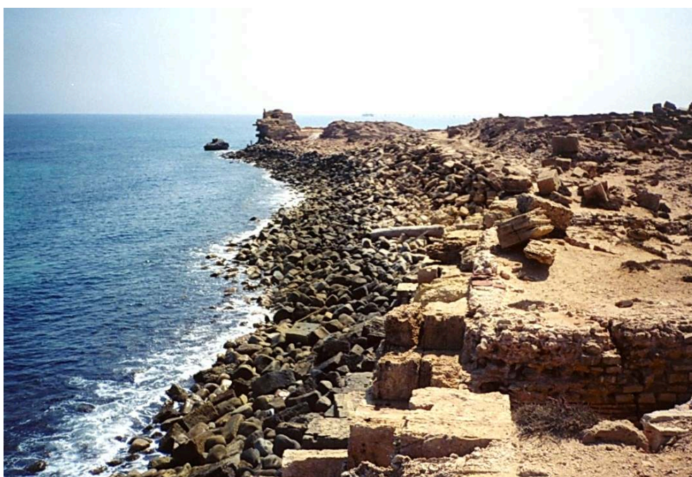
Fig. 32. Berm breakwater on the north coast of Leptis Magna
