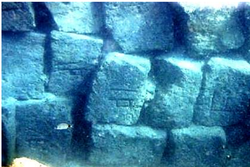
Built with ashlar headers (0.5x0.5x2 m) Noureddine, 2010
