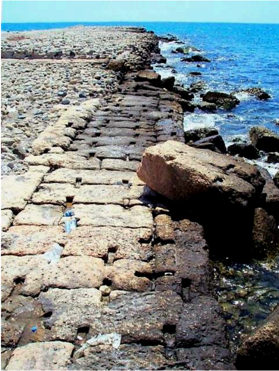
Fig. 8. Marginal ashlar wall (centre) containing marine concrete (left) at Pompeiopolis
