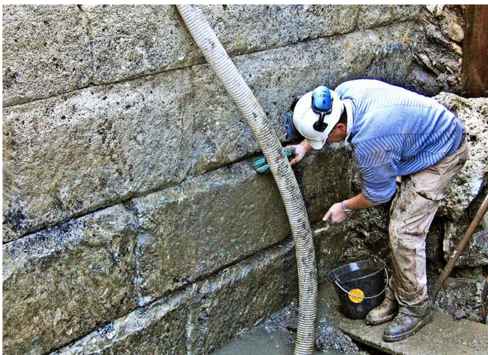
Built with ashlar stretchers Inrap, 2006
