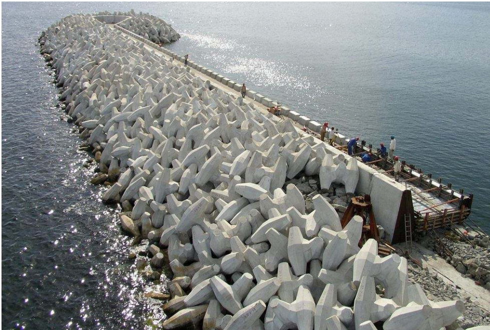
Fig. 33. Fujairah breakwater under construction (UAE)
