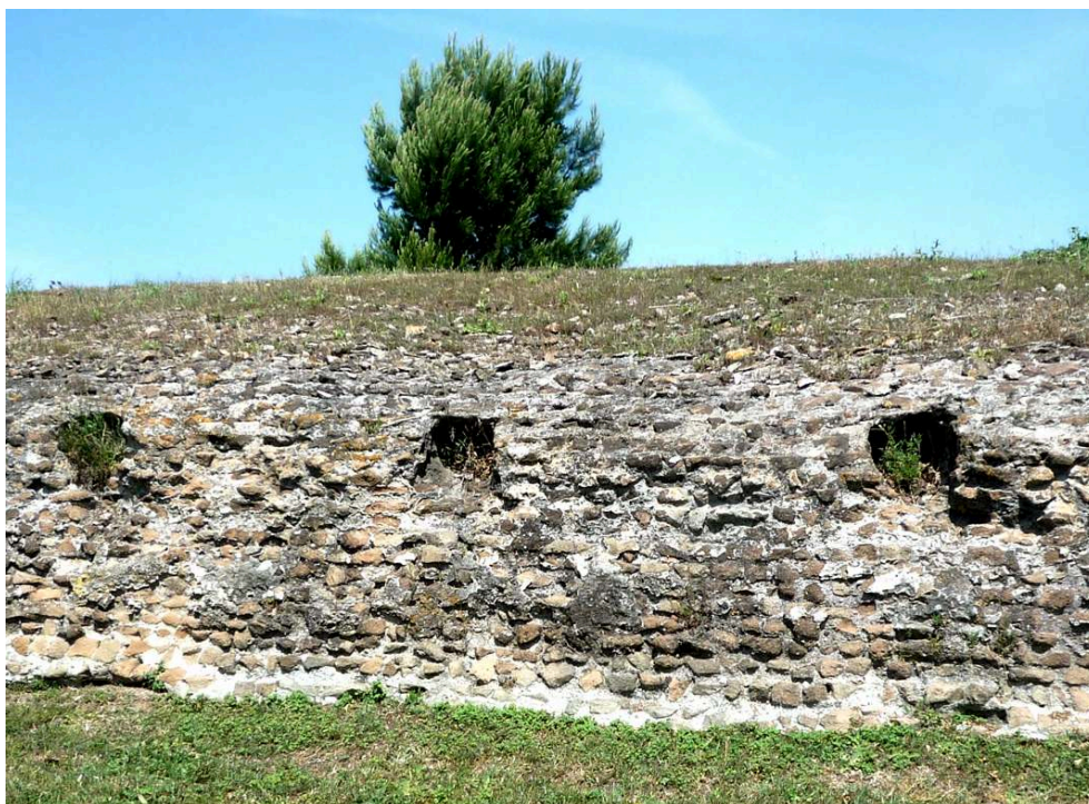
Fig. 5 - Portus' north breakwater
