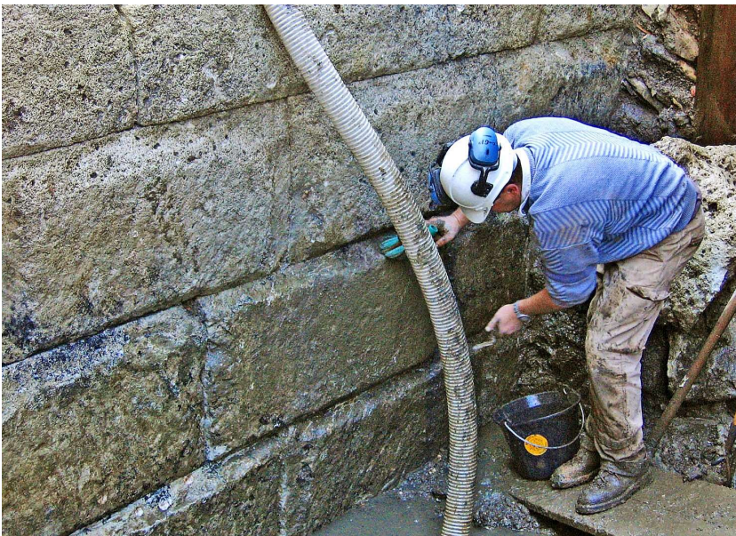
Roman quay wall at Marseille , built with ashlar stretchers (Inrap, 2006)
