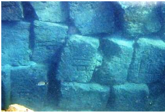
Tyre north mole built with ashlar headers, 800 BC (Noureddine, 2010)
