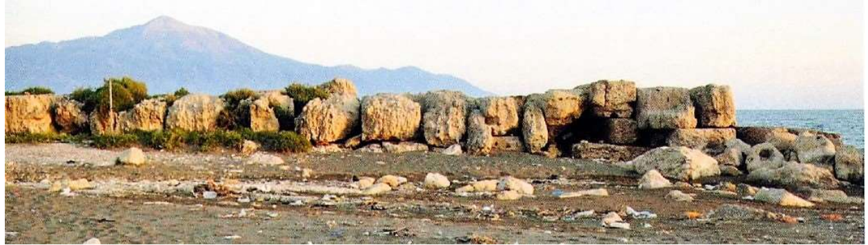
Seleucia Pieria Roman south mole built with ashlar headers, (Pamir, 2011)
