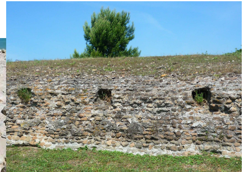
Portus' north concrete breakwater showing imprints of transverse caisson beams (Photo de Graauw, 2011)
