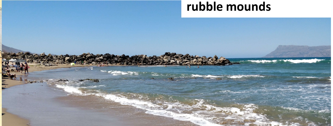
Rubble-mound breakwater at Kissamos (Crete) (Photo A. de Graauw, 2022)
