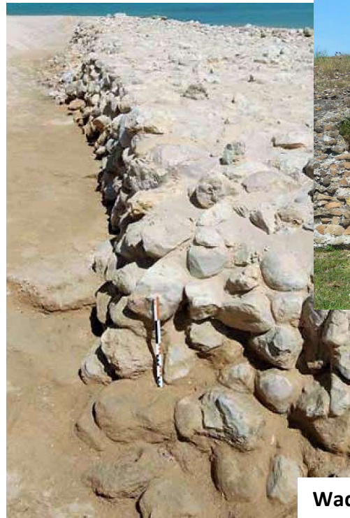
Portus' north concrete breakwater showing imprints of transverse caisson beams (Photo de Graauw, 2011)
