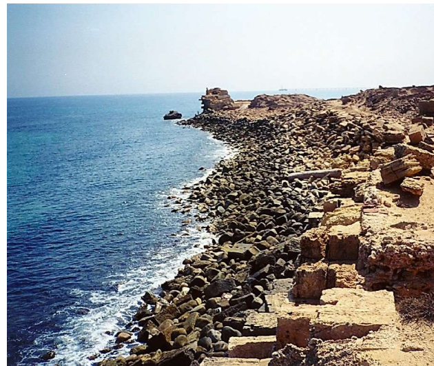
Berm breakwater at Leptis Magna (Photo A. de Graauw, 2001)
